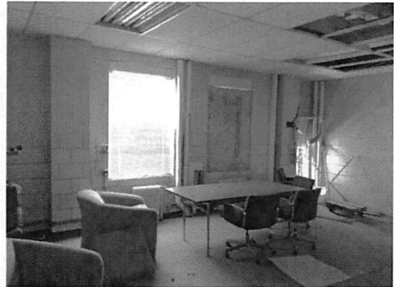
First floor office (Photo Taken on January 11, 2017)
