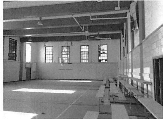
Gymnasium (Photo Taken on January 11, 2017)
